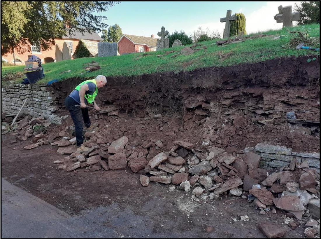
Figure 2. Dismantling of the wall using hand tools.
