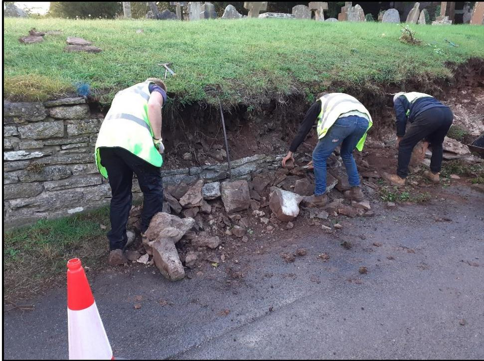
Figure 4. Work underway to dismantle the churchyard wall.
