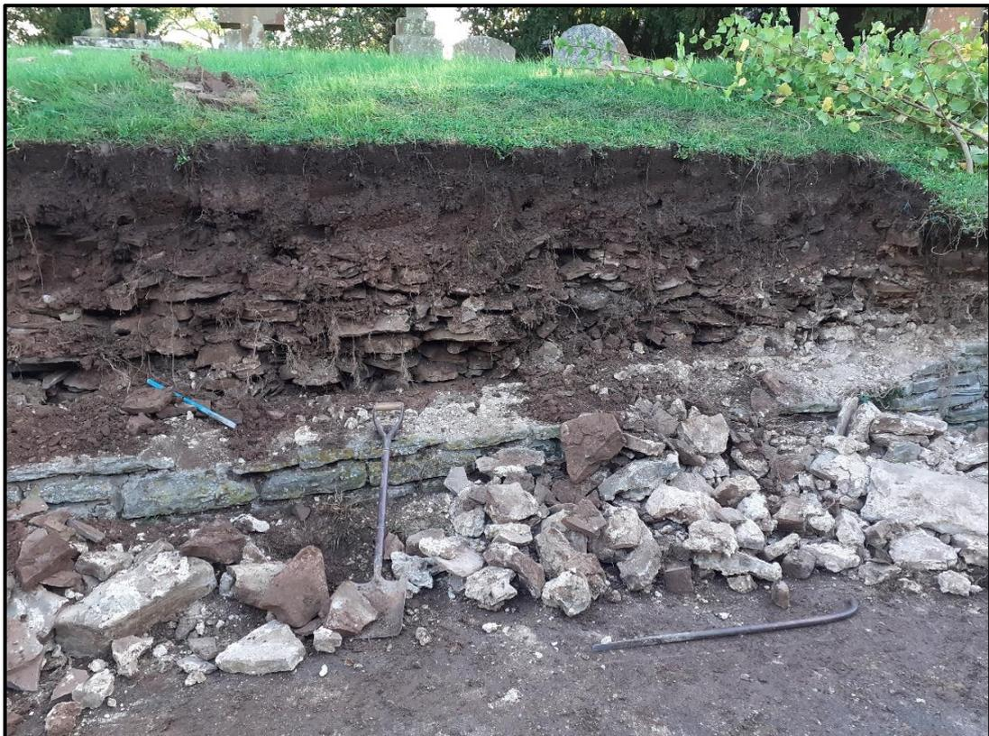
Figure 1. The exposed wall core during dismantling.
